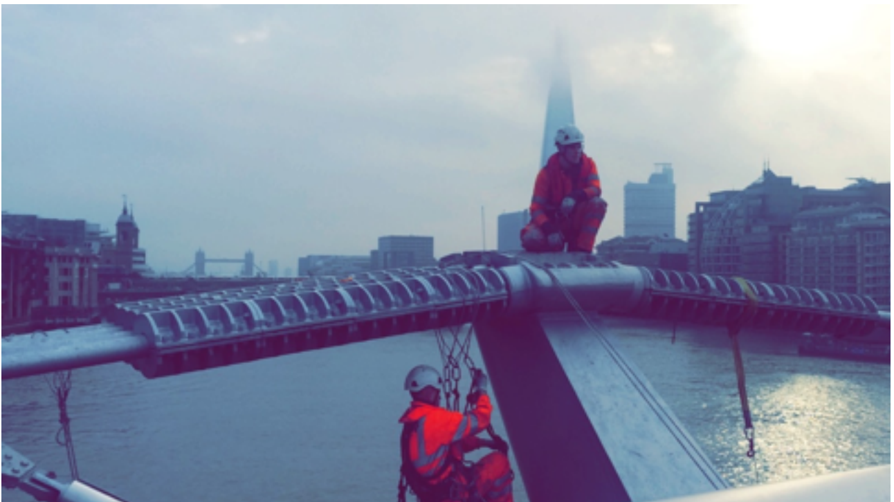
Photography by author, Construction workers working on the Millennium Bridge | November 2015
